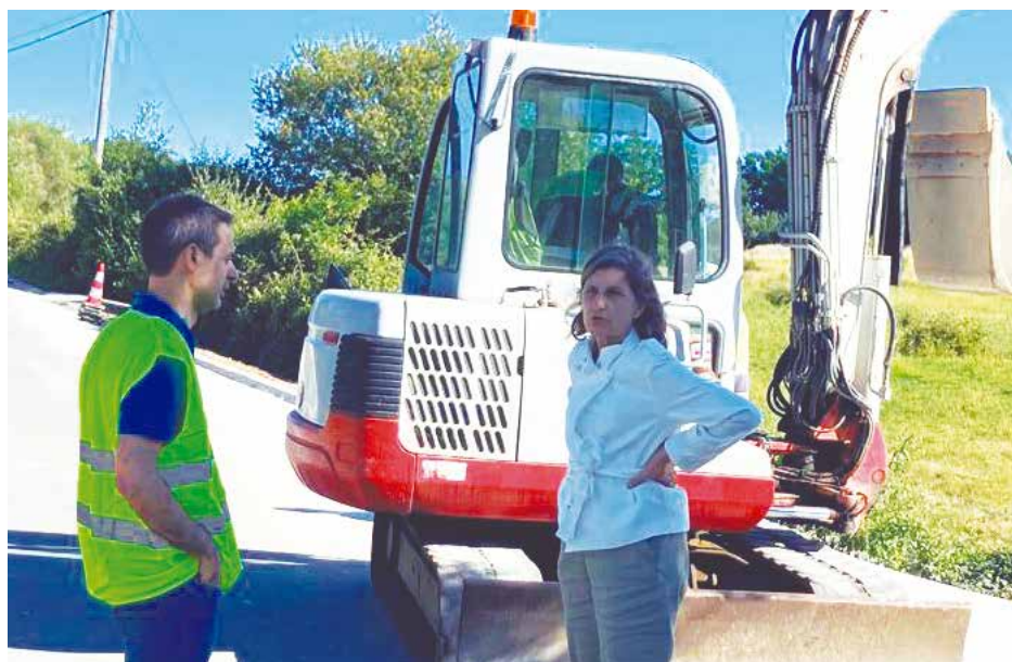
Belén Cachafeiro supervisando as obras
